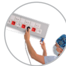
Electric cable connection
